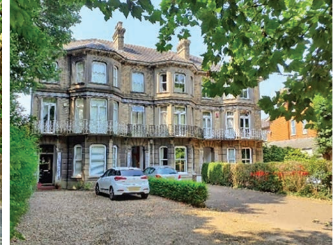
Elaborate detailing including iron balconies and railings
