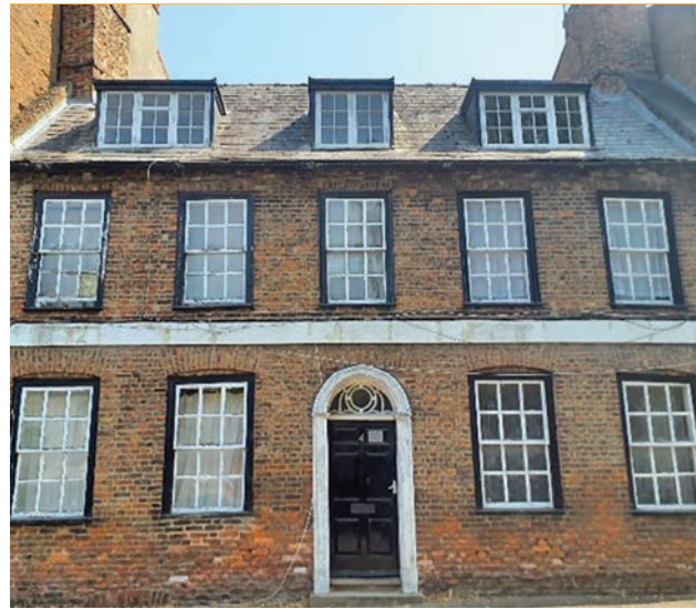
Georgian residential buildings with timber framed sash windows and dormer windows
