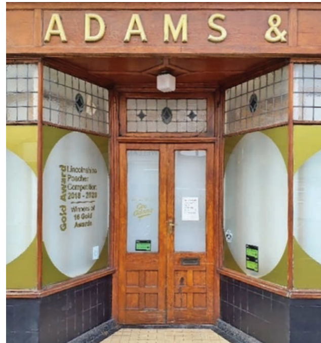
The character area contains interesting shop front features such as tiling and leaded lights
