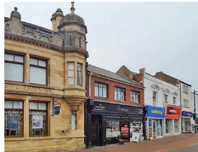
Two storey continuous facades within the Historic Commercial Centre
