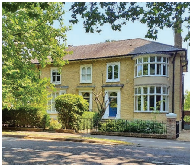
Buff brick used for residential villas along Pinchbeck Road
